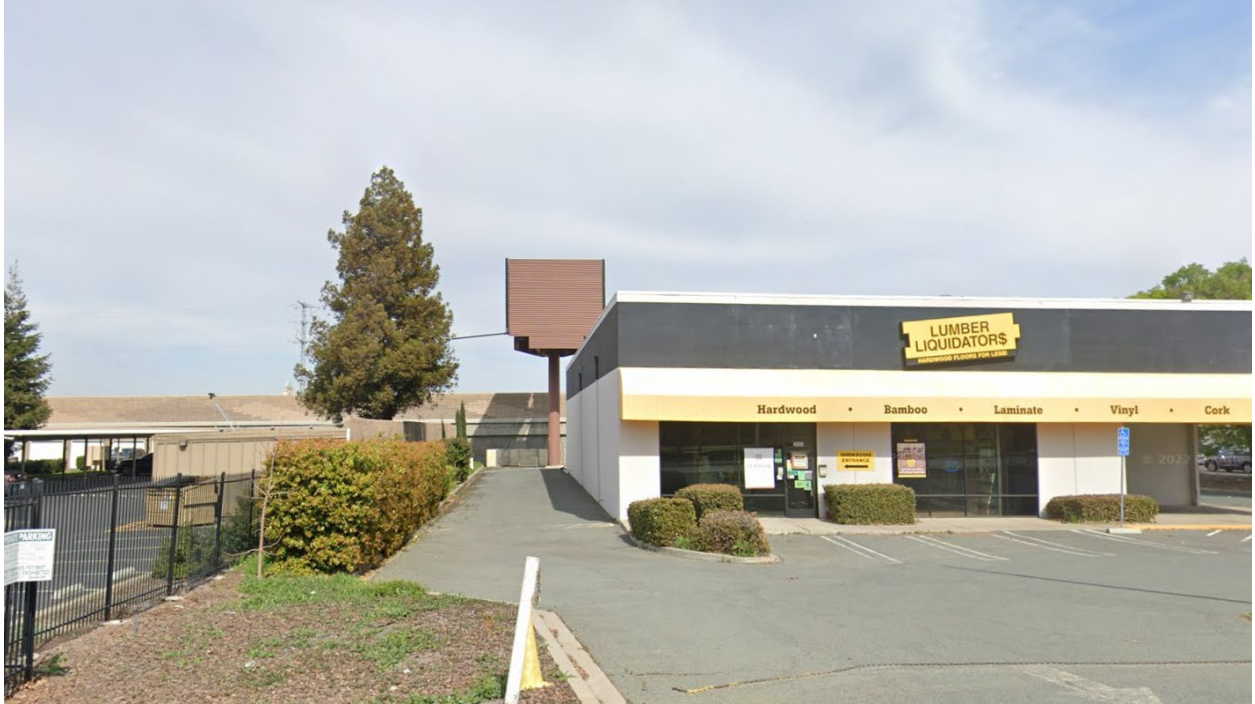
West side of subject site showing driveway exit, maneuvering aisle and parking areas
