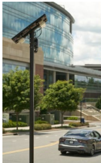
Solar & Flock Pole
