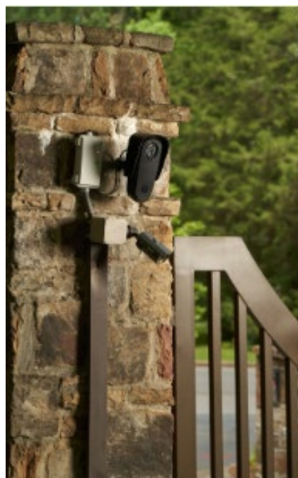
Electric & Existing Structure / Pole
